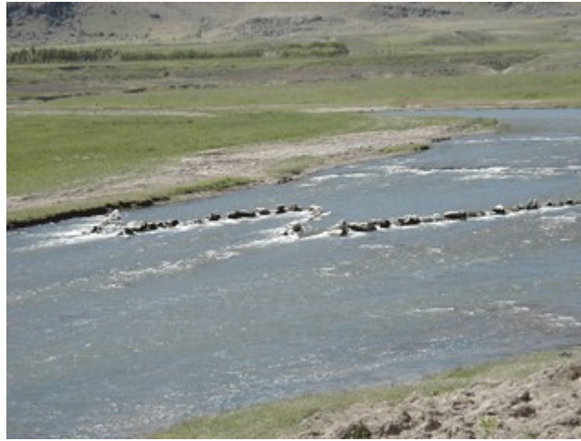
A barrier on Bendi Mahi River (Muradiye-YIBO around)
